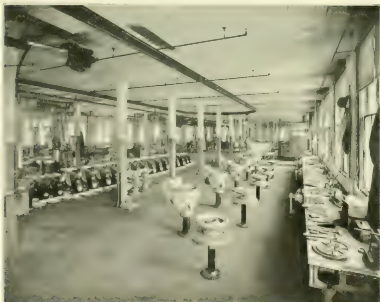
THE VALVE ASSEMBLING DEPARTMENT
