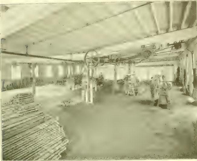
THE PIPE SHOP
