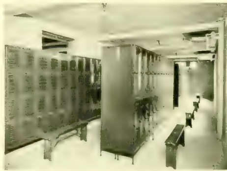
CORNER OF LOCKER ROOM
