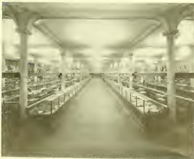
VIEW OF THE STORE LOOKING TOWARD MAIN ENTRANCE
