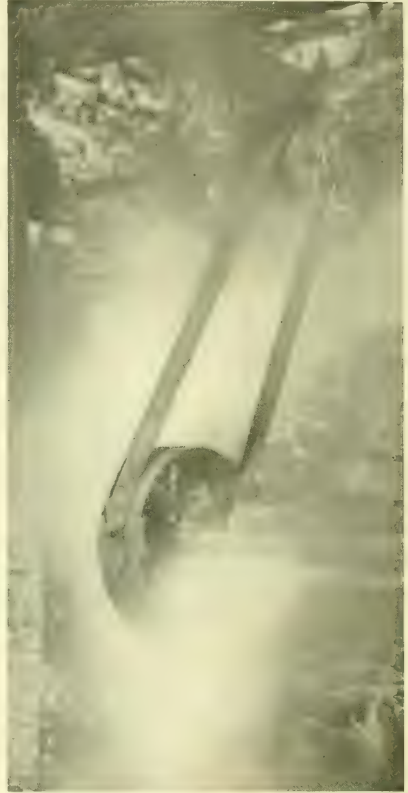
Rubber Belt at the end of SIX MONTHS' service in the same room under identically the same conditions.
