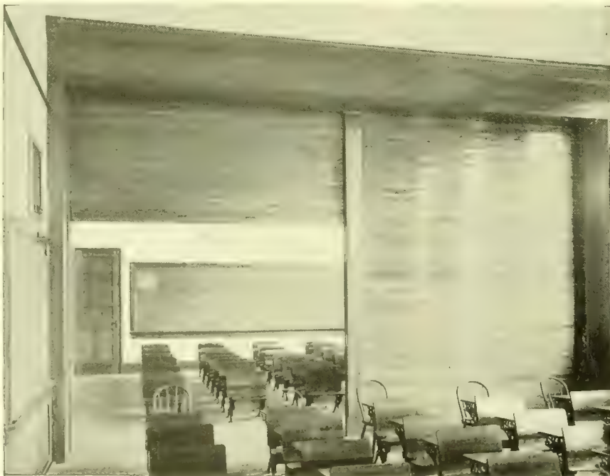
DIVISION BETWEEN CLASS ROOMS IN SCHOOL. A combination of the two rooms is obtained by a removable post
